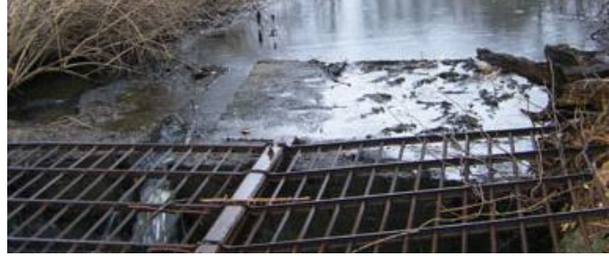
Pond Brook Circle Drainage Project
