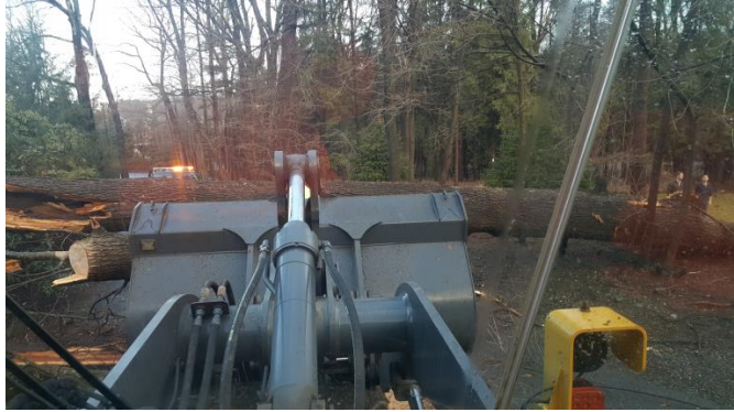
DPW employees were busy removing debris this week
