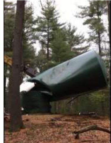
Black Oak Tank Demolition
